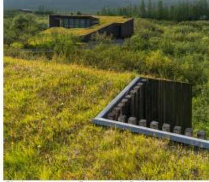
Clad containers - Green roofs & charred cladding
